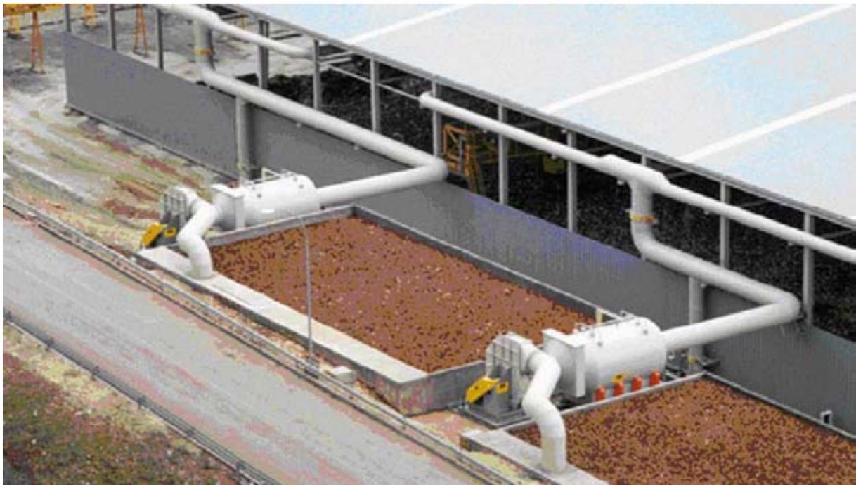
*Biofiltration Deodorization Plant, Q=72,000 m<sup>3</sup>/h y Q=50,000 m<sup>3</sup>/h; RSU treatment plant.*
