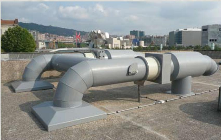
*Deodorization and Ventilation Plant  $Q=18,100 \text{ m}^3/\text{h}$ .*
